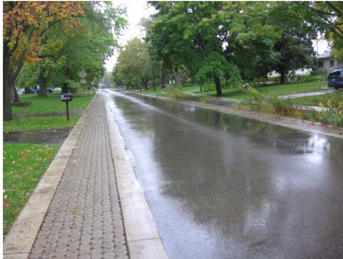
Figure 2. Easy Street re-constructed, October 2009, approximately two years after construction was completed
